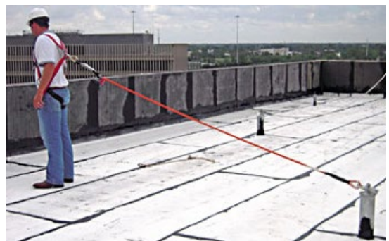
Proper use of harness w/lanyard fixed to a permanent anchor point
