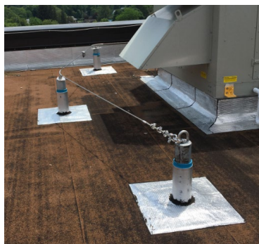
Typical permanent combination anchor point and lifeline
